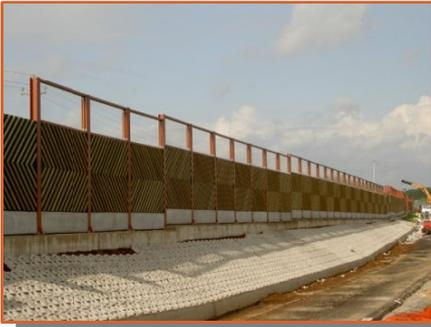
Several benefits are supposed: in addition to a high absorption capacity and to a consequent reduced acoustic reflection demonstrated by appropriate tests, the prototype can also perfectly integrate under an aesthetic point of view in the environment; therefore, it can be suitable for installation in places which require a low visual impact, like landscape or residential areas.
